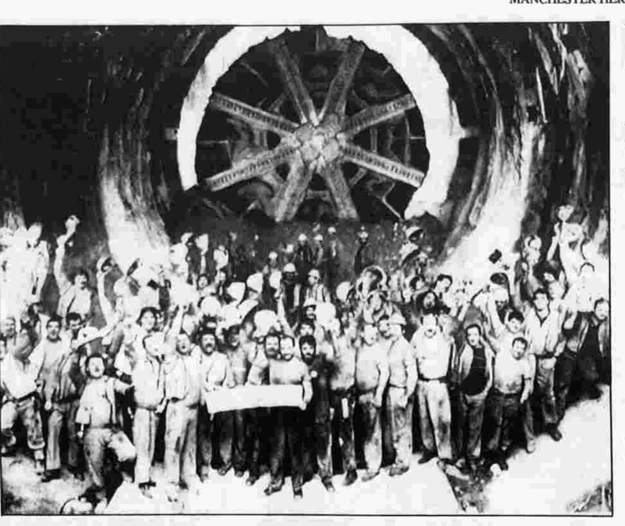
END OF LAND TUNNELLING — Channel tunnel workers celebrate their arrival in Folkestone, Tuesday, when the final underground section between the Kent coast and the terminal site broke through which signalled the end of land tunnelling.
